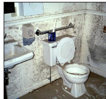
Figure 1-15 Mold and mildew can grow quickly after a flood
