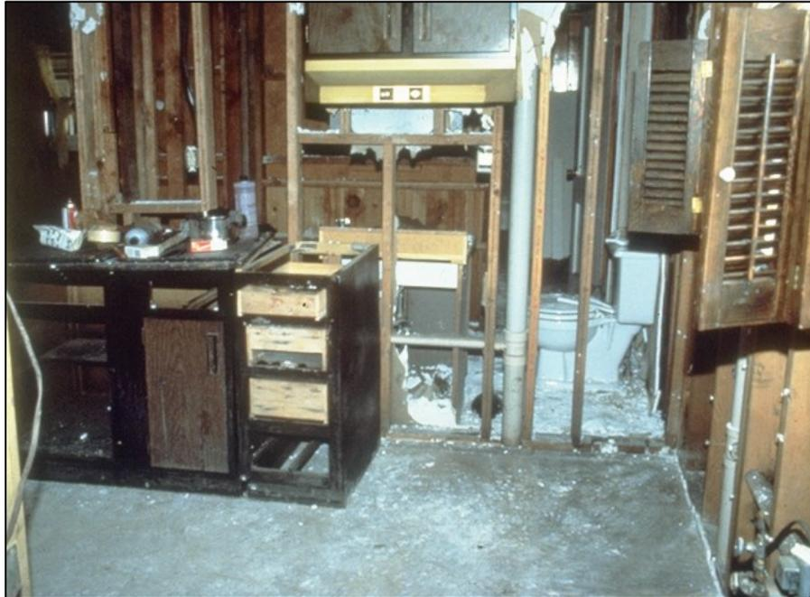
**Figure 12-15 Even slow moving floodwater can cause substantial damage**
