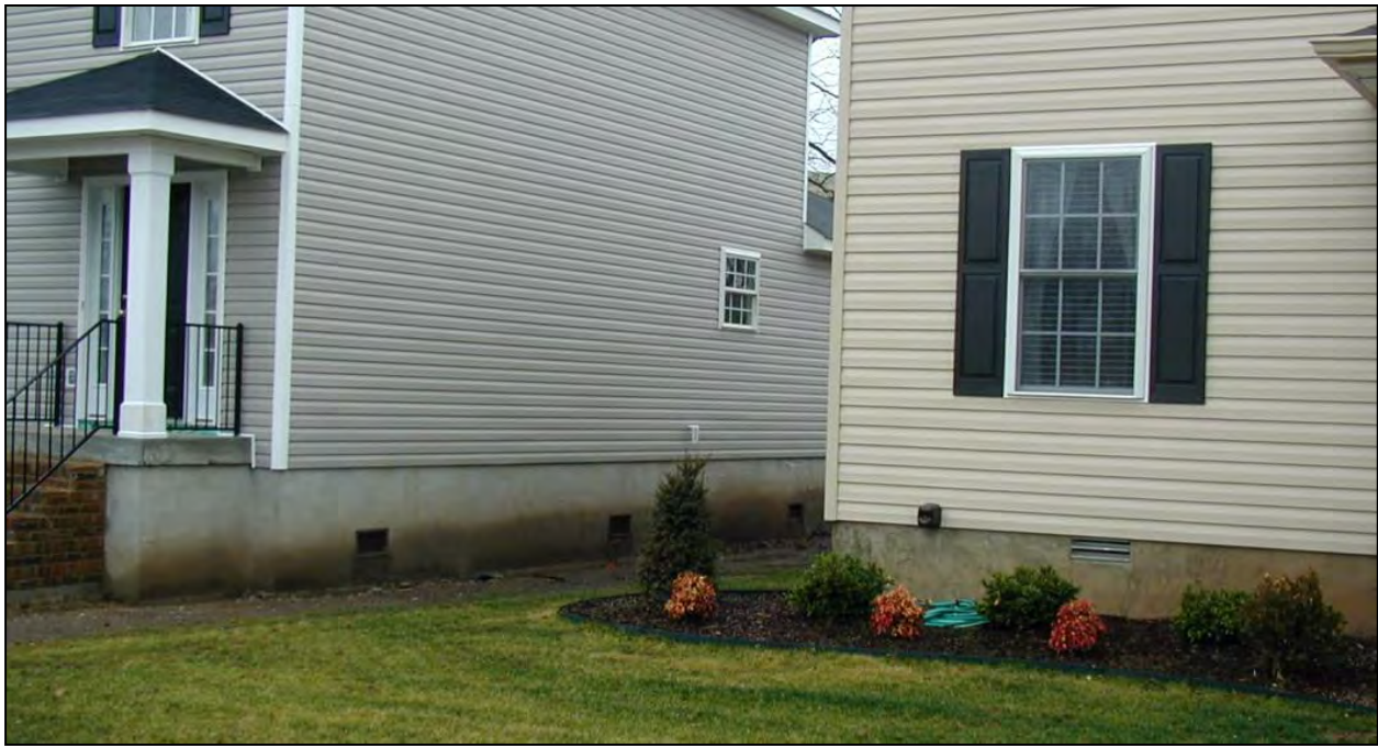
Figure 11-8. The house on the left has compliant crawlspace openings. The openings in the foundation on the right are too high.
