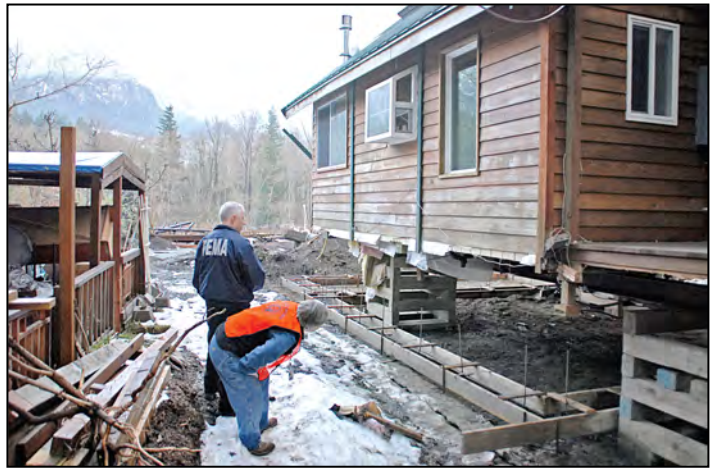
Figure 12-17. In-process elevation project to bring a substantially damaged building into compliance
