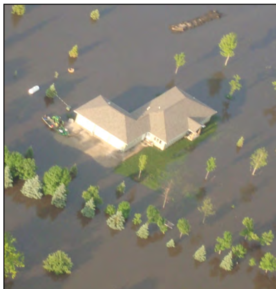
Figure 11-1. A new building elevated on fill plus freeboard was not damaged by this flood
