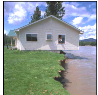
Figure 1-6. Riverine erosion can undercut structures
