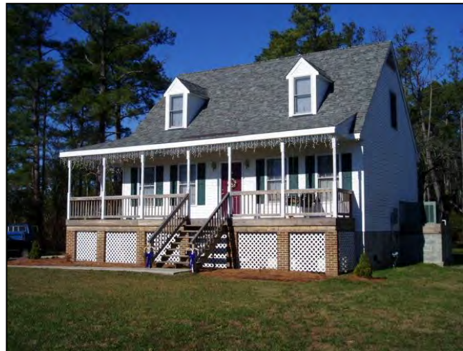
Figure 11-3. Building elevated on crawlspace with foundation openings
