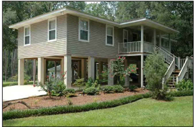
Figure 11-2. Structure elevated on piers
