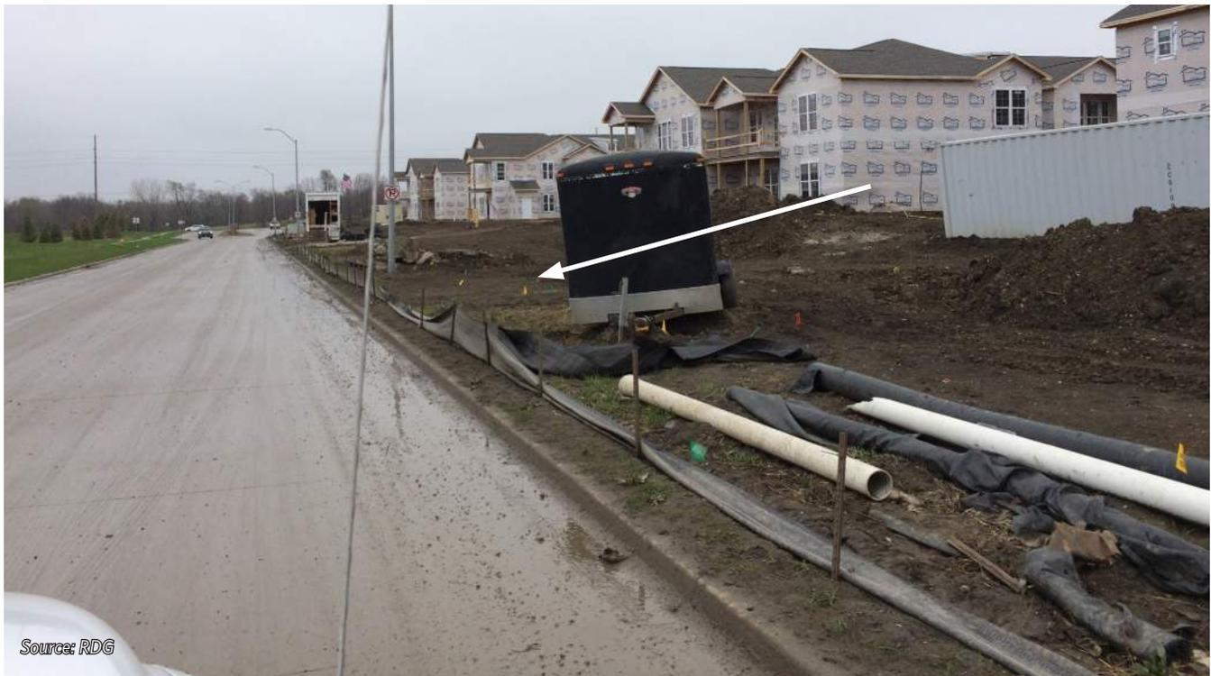
Tracking from a construction site onto a paved roadway from an unprotected construction entrance.
