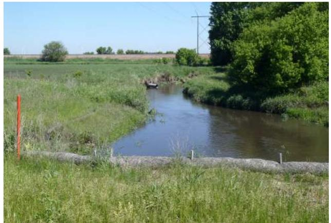
Bank movement has left this tile outlet projecting into the stream in the Beaver Creek watershed.
