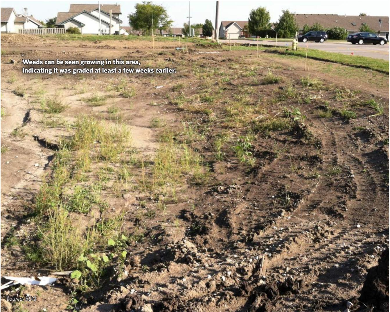
This area has not been seeded or mulched, leaving it exposed to potential erosion.
