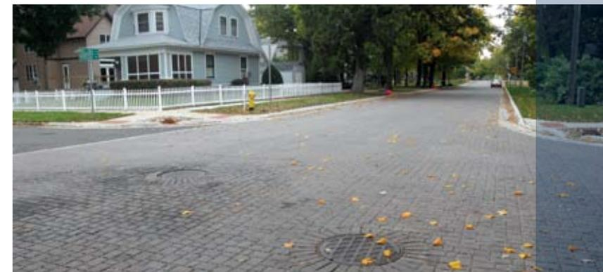
*Permeable pavers help soak up and filter runoff from rain and snow.*
