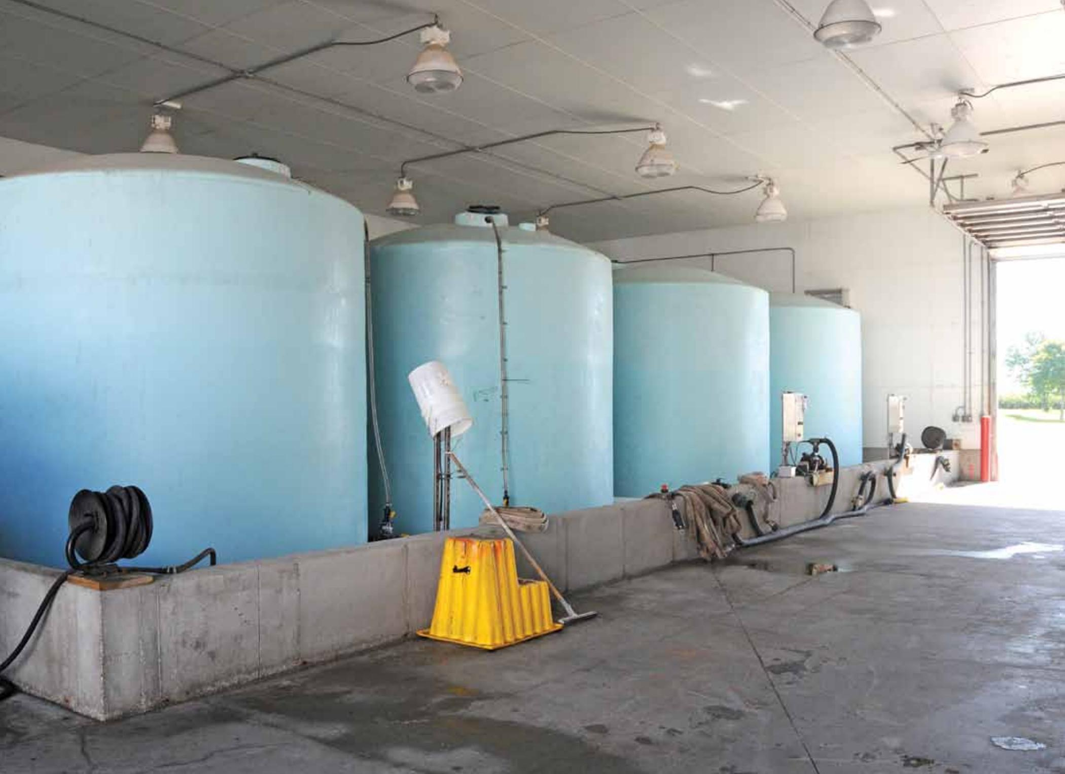
*Wash water collected at DOT truck washes is filtered to remove oil and grit, then mixed with salt to create brine for treating roads in winter driving conditions.*
