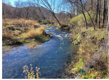
created floodplain bench and all the reshaped streambanks. The floodplain bench will provide anglers easier access to fishing locations along the stream and also provide a serviceable floodplain during high flow seasons.
