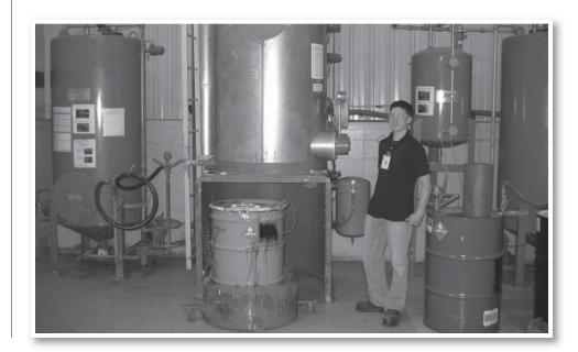
conversion of the single pass system to a recirculation loop will reduce the amount of water consumed by the distiller to almost zero and in the process reduce the total amount of water used at Vermeer by 12 percent.
