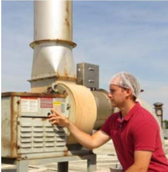
certain specifications. The estimated rate of energy leaving the facility through the 53 exhaust stacks is 180.5 therms per hour. Capturing this thermal energy could provide opportunities to reduce natural gas usage in other areas of the plant such as heating water and intake air and help achieve a closer air balance in the plant.
