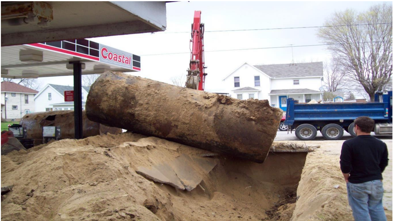
Tank removal in Waukon. Planning a tank removal must consider overhead power lines and canopies that can present risks for removers. Please note, the person standing close to the excavation is not wearing safety equipment and the excavation is not barricaded.
