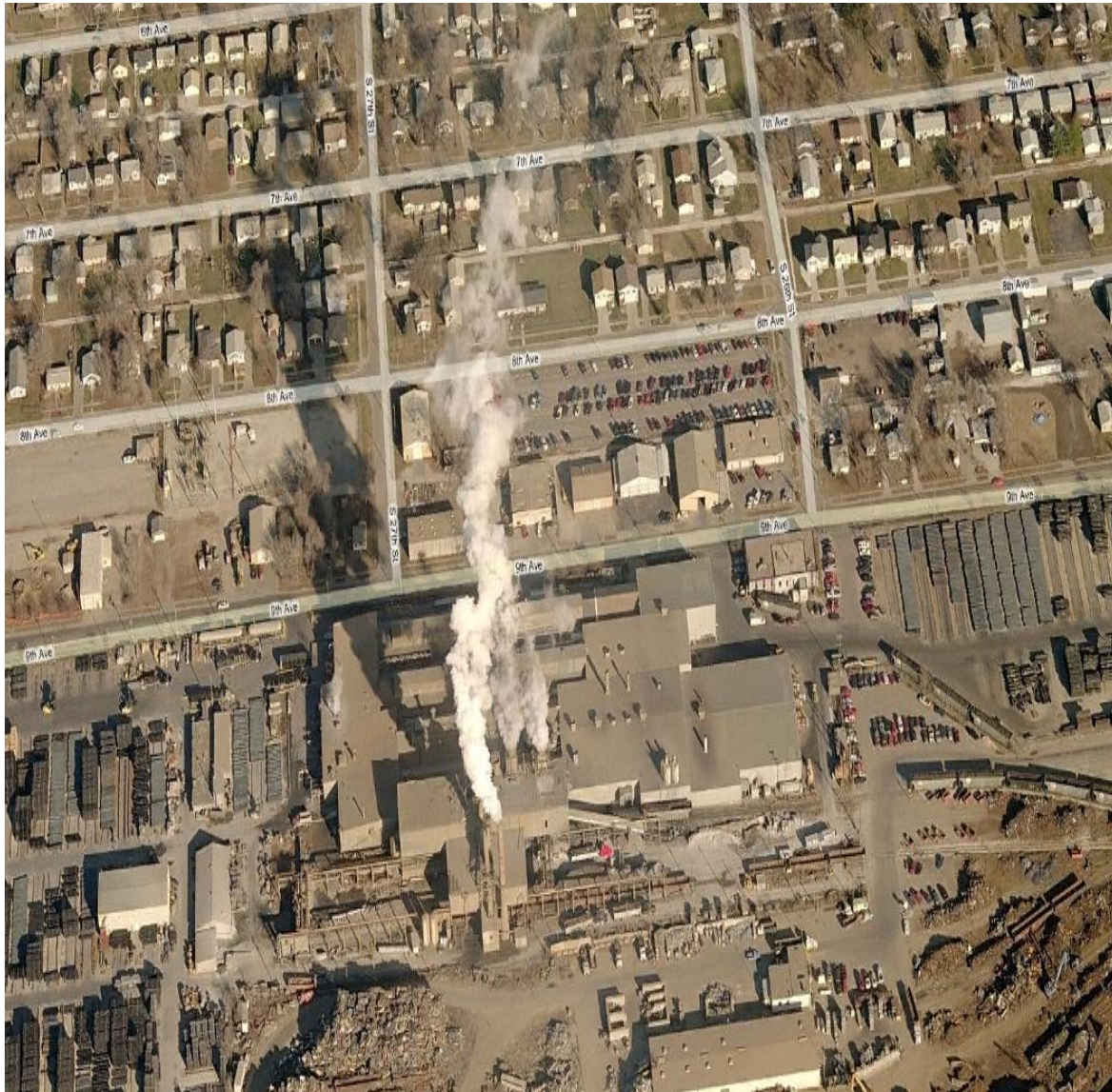
Figure 1. Aerial view of Griffin Pipe Products Company and some of the adjacent properties (mostly residential) to the north. 12
