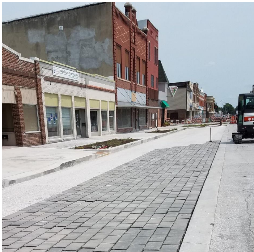
Figure 58: Permeable Pavers in Eagle Grove, Designed to Treat Urban Stormwater Runoff
