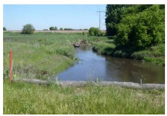
Bank movement has left this tile outlet projecting into the stream in the Beaver Creek watershed.
