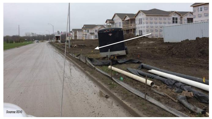
Tracking from a construction site onto a paved roadway from an unprotected construction entrance.
