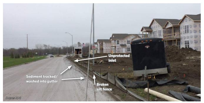
Perimeter controls that have not been maintained that are allowing sediment to be washed into the street gutters and storm sewers.
