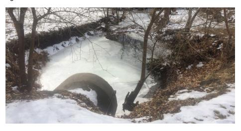
Figure 9.10-1-11-A: Level spreader outlet structure
