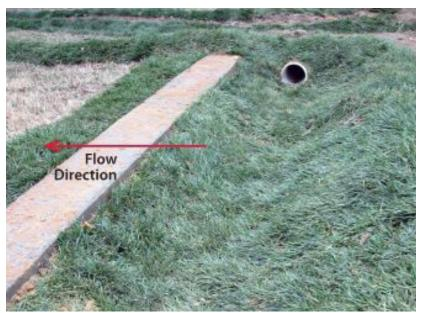
Concrete level spread with grass basin on upstream side. Flow enters from pipe that runs parallel to the spreader and leaves by filling the basin and flowing across the level concrete strip. (photo coutesy - NC State University "Urban Waterways - Level Spreader Update")
