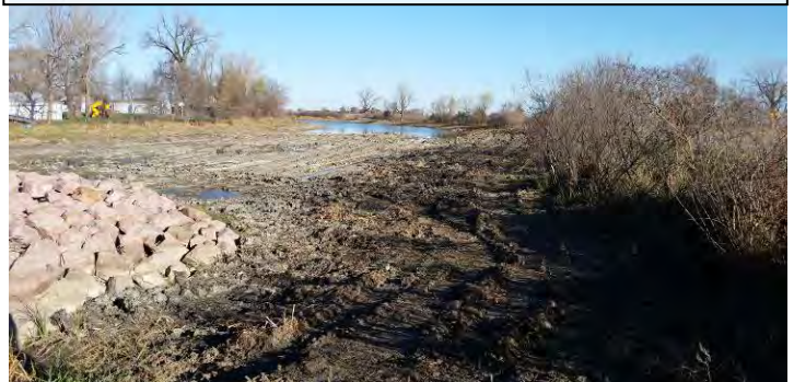
Completed construction on Nebowa Bay in Fall 2016
