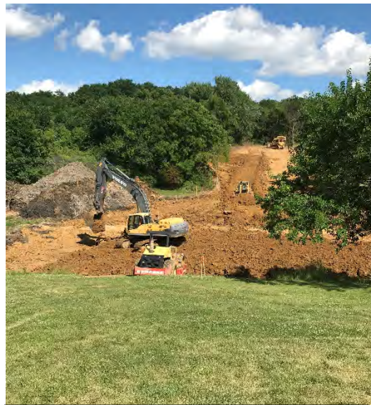
Construction at one of the watershed ponds constructed in the part as a part of the restoration efforts.
