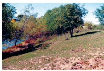
spillways, as root systems provide seepage paths for water, especially after roots decay. Trees that fall over or are blown down can leave large holes in the embankment surface. weakening the embankment and
