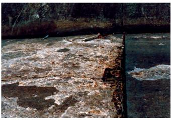
Concrete deterioration has exposed reinforcing steel and created a hole in the chute spillway floor above.
