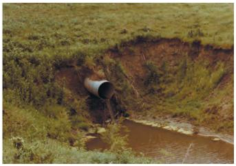
Erosion of an outlet channel.
