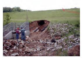
Piping failure of a dam as a result of seepage along the spillway conduit. A hole has eroded completely through the dam.
