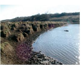
Excessive erosion on an upstream slope, due to grazing cattle and wave action.
