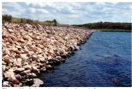
waterline, forming a beach or **berm**. The deposition is not harmful, but the eroded cavity above the water line steepens a front slope and weakens the upper embankment. Carried to an ultimate result, the embankment would be destroyed.
