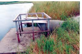
A typical concrete pipe hood inlet spillway with antivortex plate, trash rack and scour pad.
