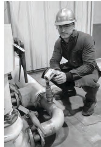
**Direct Steam Injector PM:** CCC has an onsite wastewater treatment plant. During the cooler months, a direct steam injection (DSI) system keeps the influent heated to a temperature where the microbiological organisms can function efficiently. DSI heaters benefit from preventative maintenance (PM) plans, which keep them operating efficiently by preventing excessive steam use and relieving stress on
