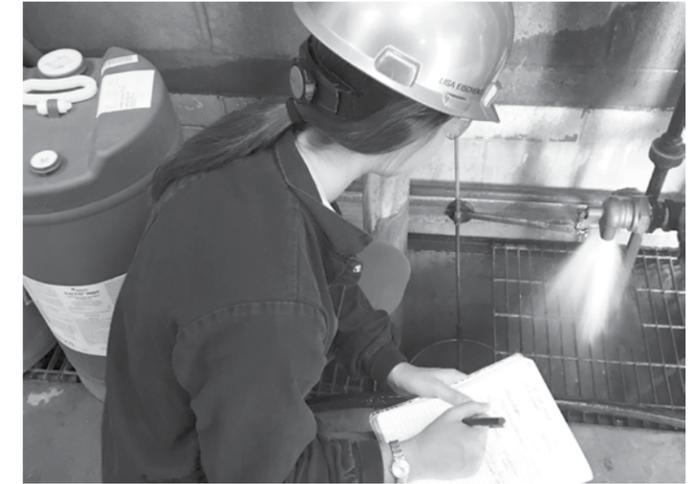
**Pipe Insulation:** Steam and condensate piping was traced in two production work centers. Maps were created and provided to a contractor to install new pipe insulation where previous insulation was missing or damaged. Insulation is necessary on all steam and condensate pipes to protect employees in work areas, and to reduce energy losses.
