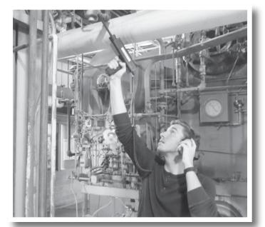
**Trap Repair & Replacement:** During the audit there were several steam traps identified that had failed and should be replaced to reduce steam loss. This would significantly reduce the amount of steam produced because the steam would be used more effectively instead of being wasted. With less steam generated, the total amount of emissions produced from the boilers would decrease as well.
