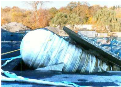
Tank floating out of ground, Rockaway River, NJ
