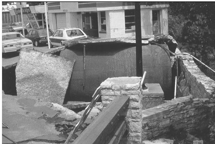
UST lifted by buoyant force
