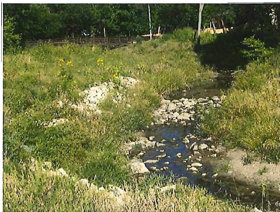
Photo 2 – After completion of Yeader Creek Phase 1 (Looking upstream at SW 12 th St. pedestrian bridge)
