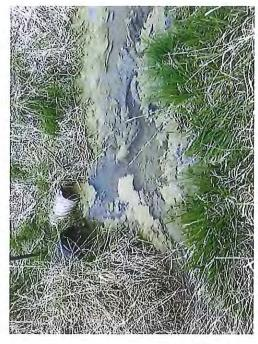
Photo 16, Black tile from Walz Energy. Precipitated silt in and around the Walz tile outlet.
