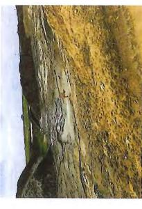
Photo 12, Red tile riser in the southwest portion of Walz Energy site. Note no tile sock or rock around
