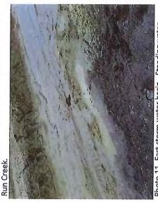
Photo 11, East storm water basin. Standing water appears to have soaked into the tile.
