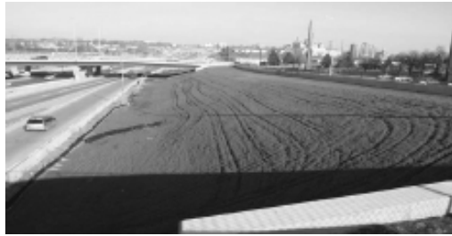
Established vegetation along the I-235 corridor helps maintain this slope.
