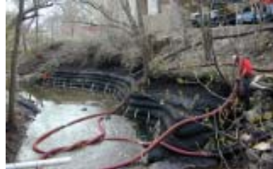
Application of compost at ISU to stabilize stream near a parking structure in April 2004
