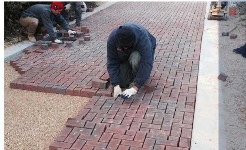
*Workers install a permeable paver system in Clinton.*
