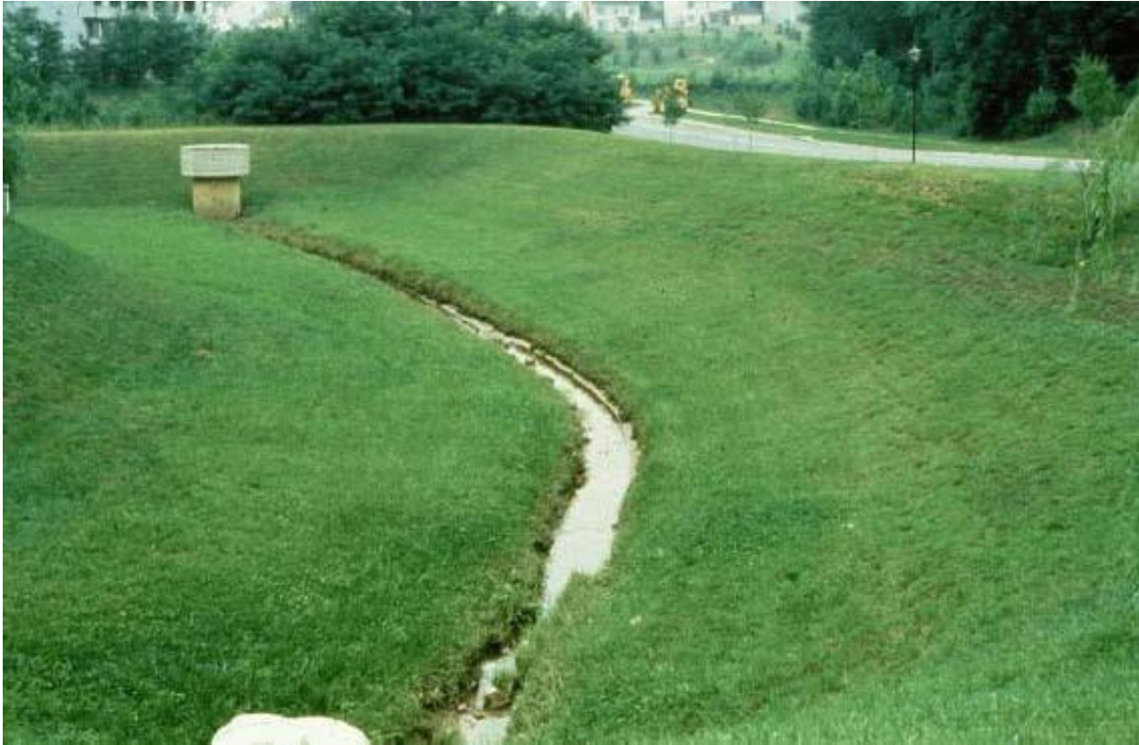
Figure C7-S1- 1: Dry detention basin
