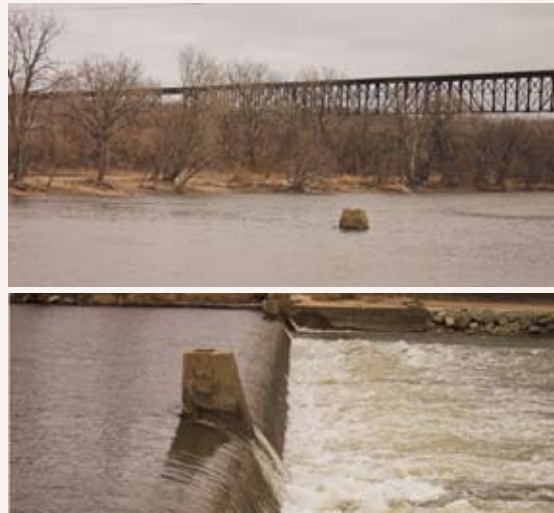
Hard to see. Falling a few feet, Little Dam in Fort Dodge can be difficult to see from upstream. From the side, its danger is readily apparent.
