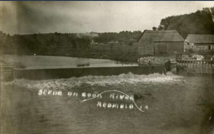
The Redfield Dam on the Middle Raccoon River.
