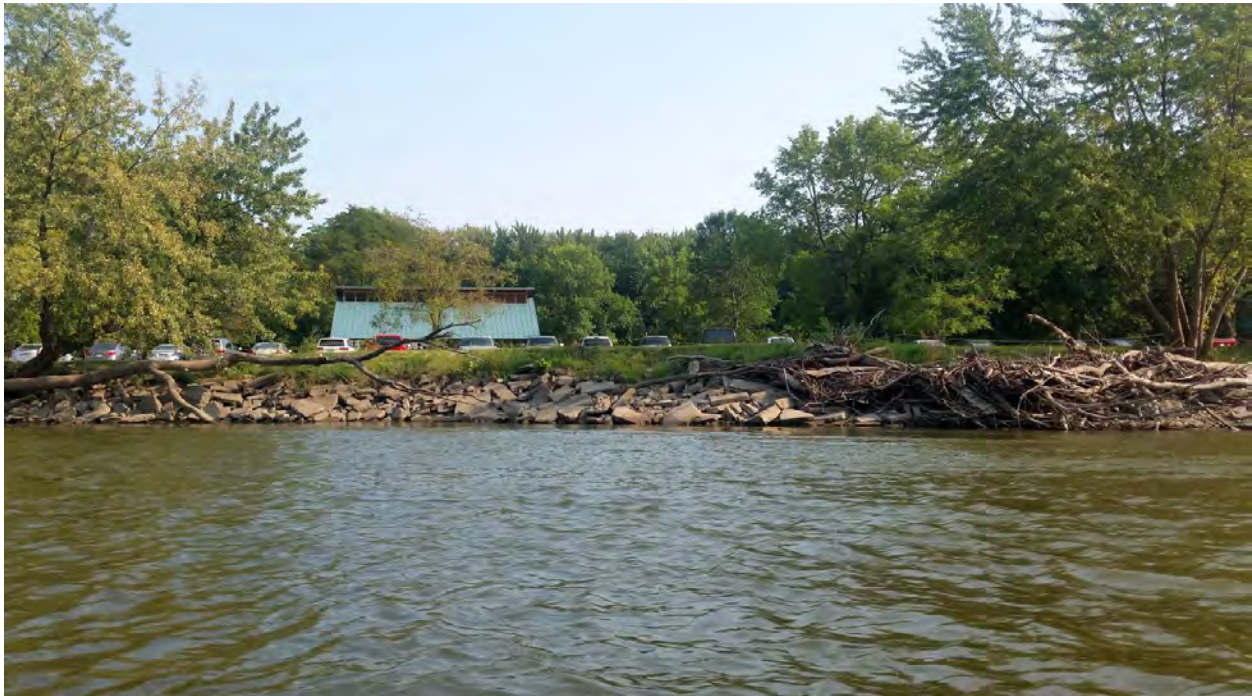
Streambank conditions near Black Hawk Park boat ramp and Riverview Shelter
