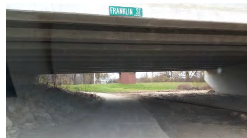
Existing trail under Center St/Franklin St Bridge
