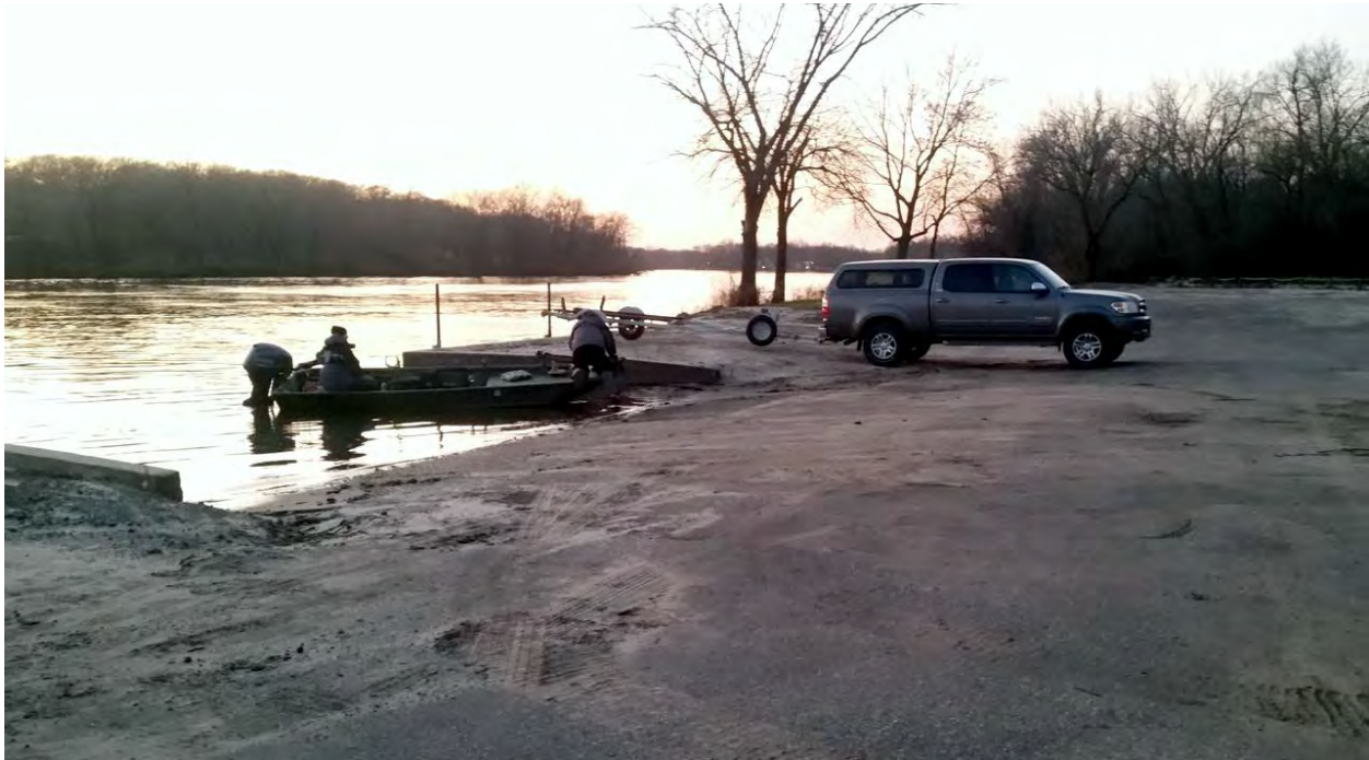
Existing motorized boat ramp at Island Park
