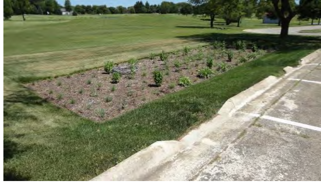
Bioretention cell installed in Cedar Falls as part of the Dry Run Creek Watershed Improvement Project Photo: Black Hawk Soil and Water Conservation District
