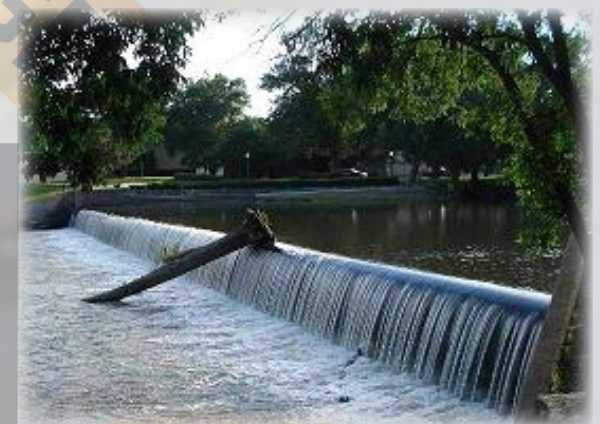
The Alden Dam on the Iowa River, in Alden, IA where two canoeists died on April 29, 2007.
